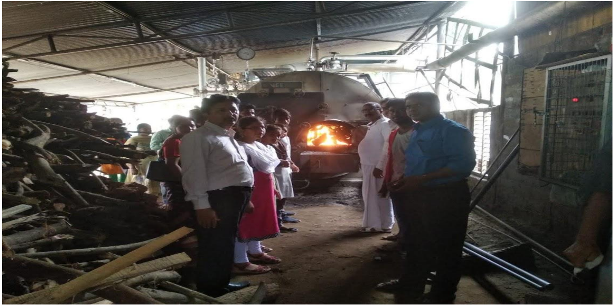
At Fire Boiler
